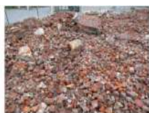
Brick and concrete waste from the partial demolition
